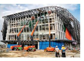
ABOVE AND RIGHT: The electric glass attachment boom lifts are powered by 80-V, 520-Ah maintenance-free high-capacity lithium battery pack with quick charging of 1.5 hours.
